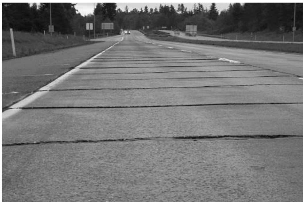
Figure 7: Example of Faulting
