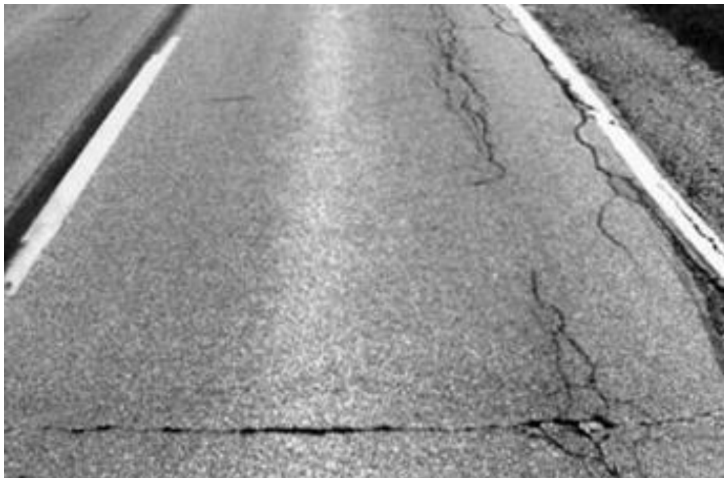
Figure 8: Example of Cracking
