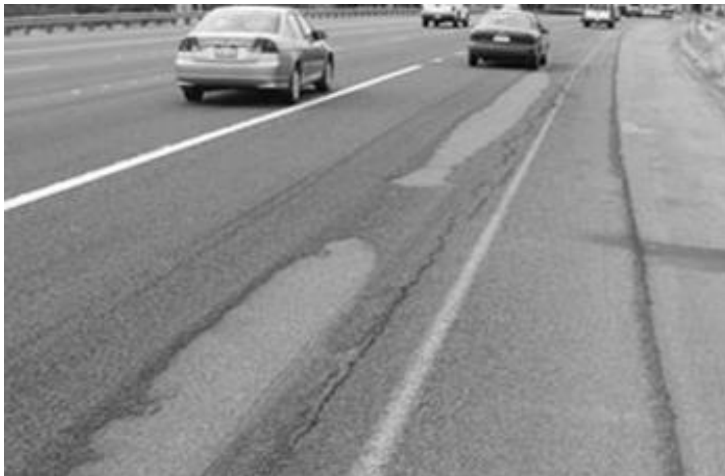
Figure 6: Example of Rutting
